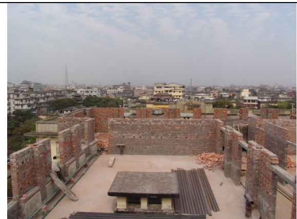
The new wing on the roof under construction
