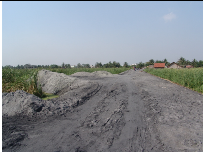
Land for 2 nd campus along Eastern Metropolitan By-pass
